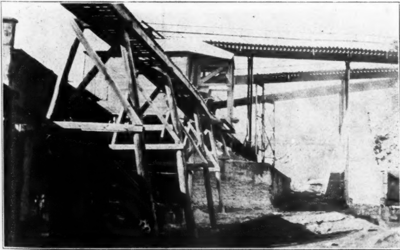
Tracks Leading to Top of Kilns
